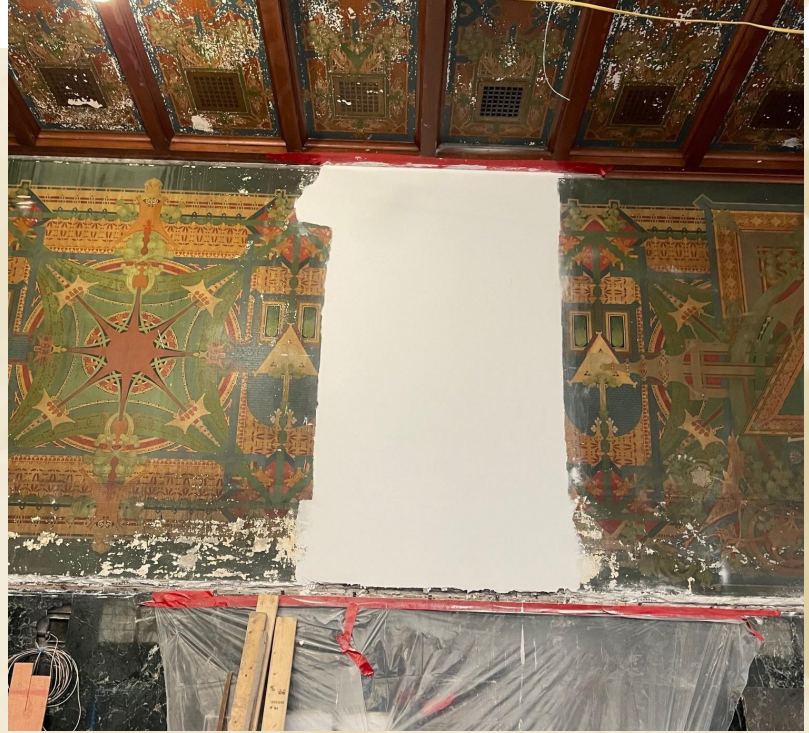
Plaster repair to make the murals restoration-ready!
